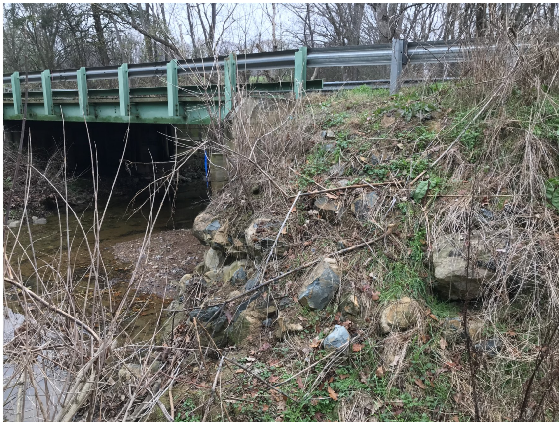
PHOTO 3: BOULDER FILL AT EB-2.
