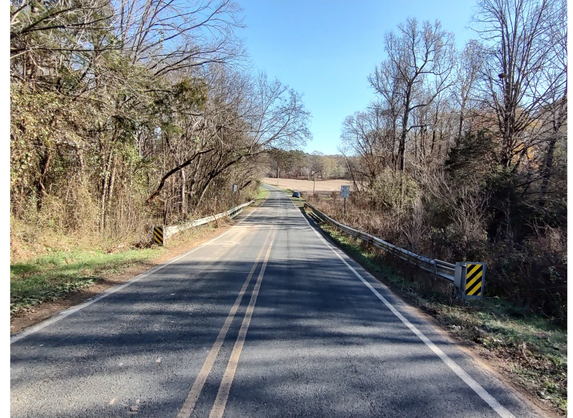
PHOTO 2: VIEW FACING BRIDGE 048 FROM -L- ALIGNMENT, FACING UPSTATION.
